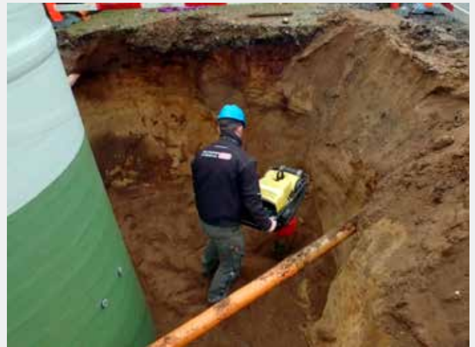
Fig. 19 Compacted layers of maximum 50 cm
