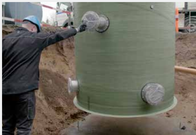
Fig. 16 Lowering the pit
