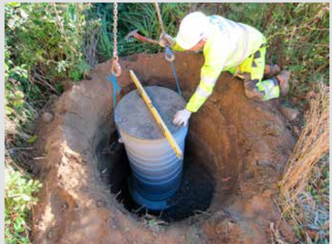
Fig. 4 Grundfos prefabricated pumping station for outdoor installation
