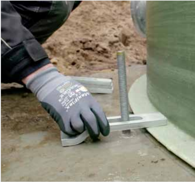
Fig. 18 Placing the mounting brackets
