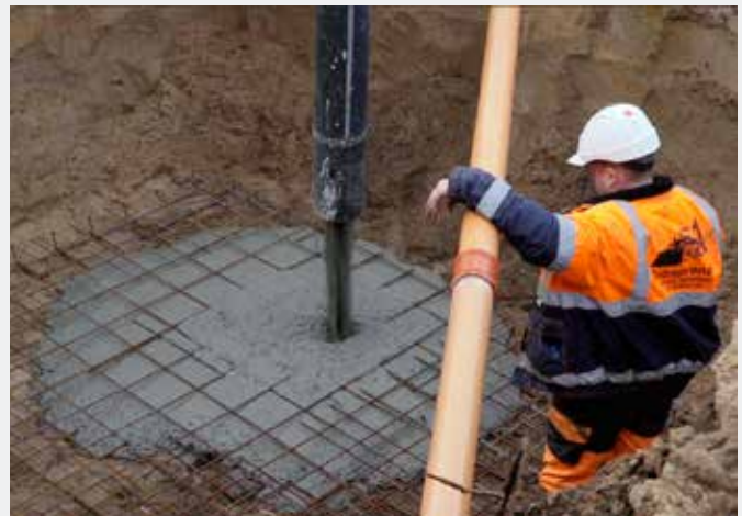
Fig. 14 Pouring of concrete slab on site
